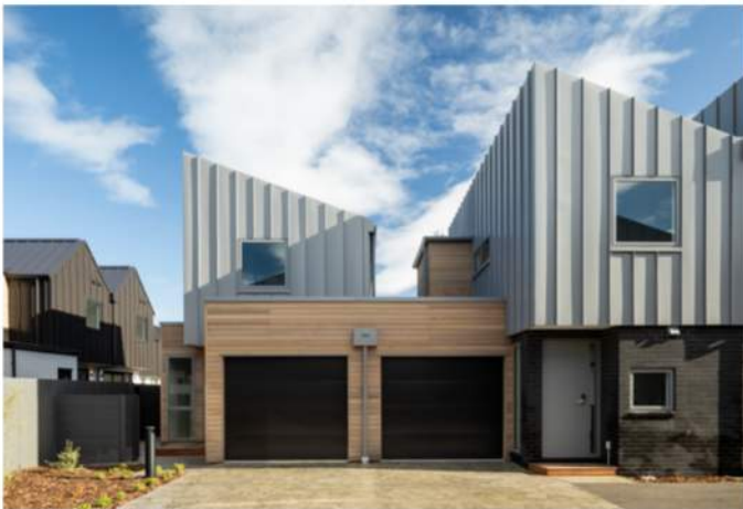
All of our homes come with either garages or dedicated parking spaces, as well as bike storage and security lighting.
